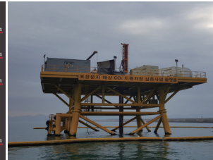
Offshore drilling for CO 2 injection
