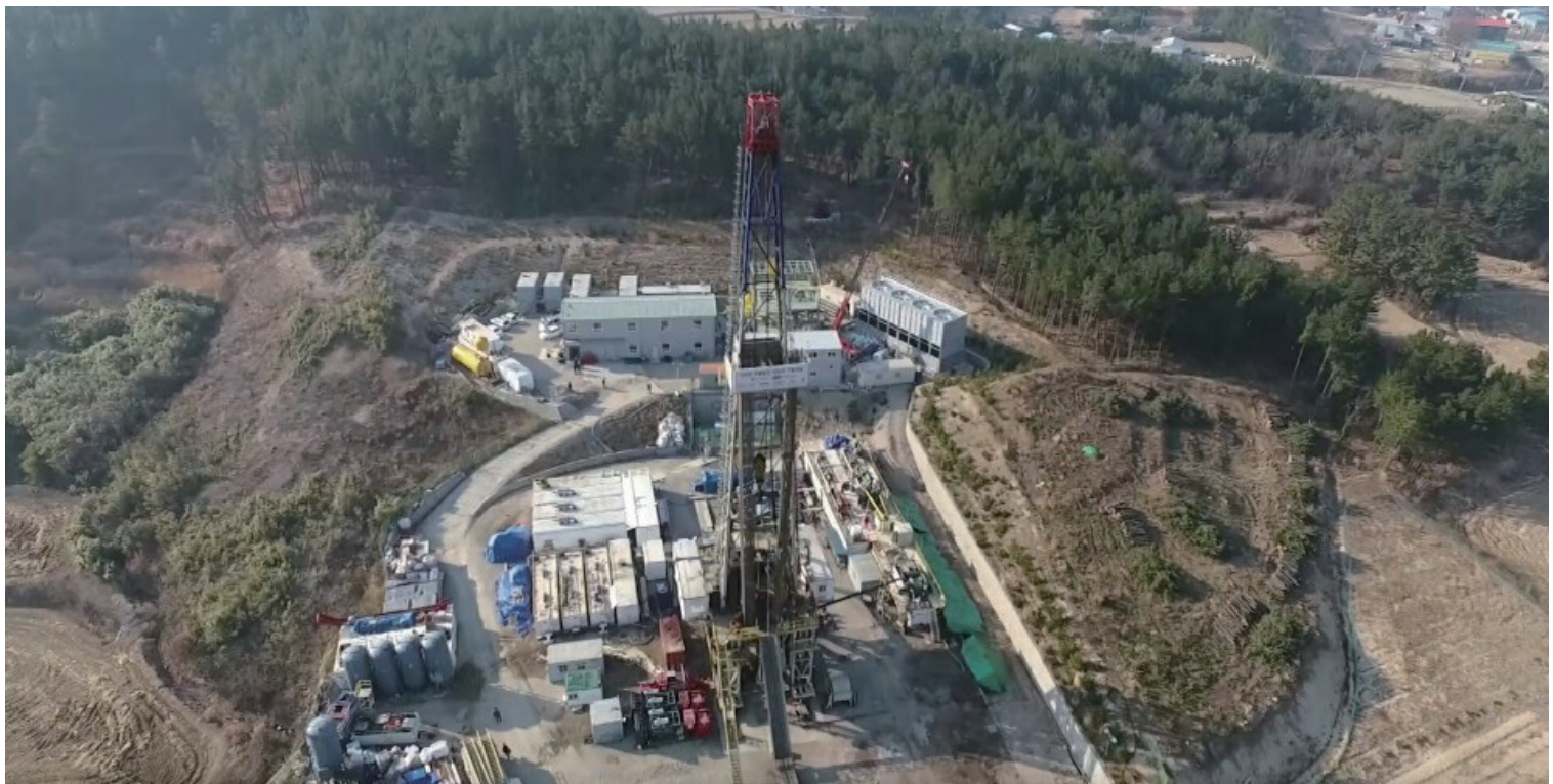
MW Scale geothermal power plant at Pohang, Southeast Korea 2 geothermal wells, PX-1 and PX-2, were terminated at 4,362 m and 4,348 m in depth respectively.
